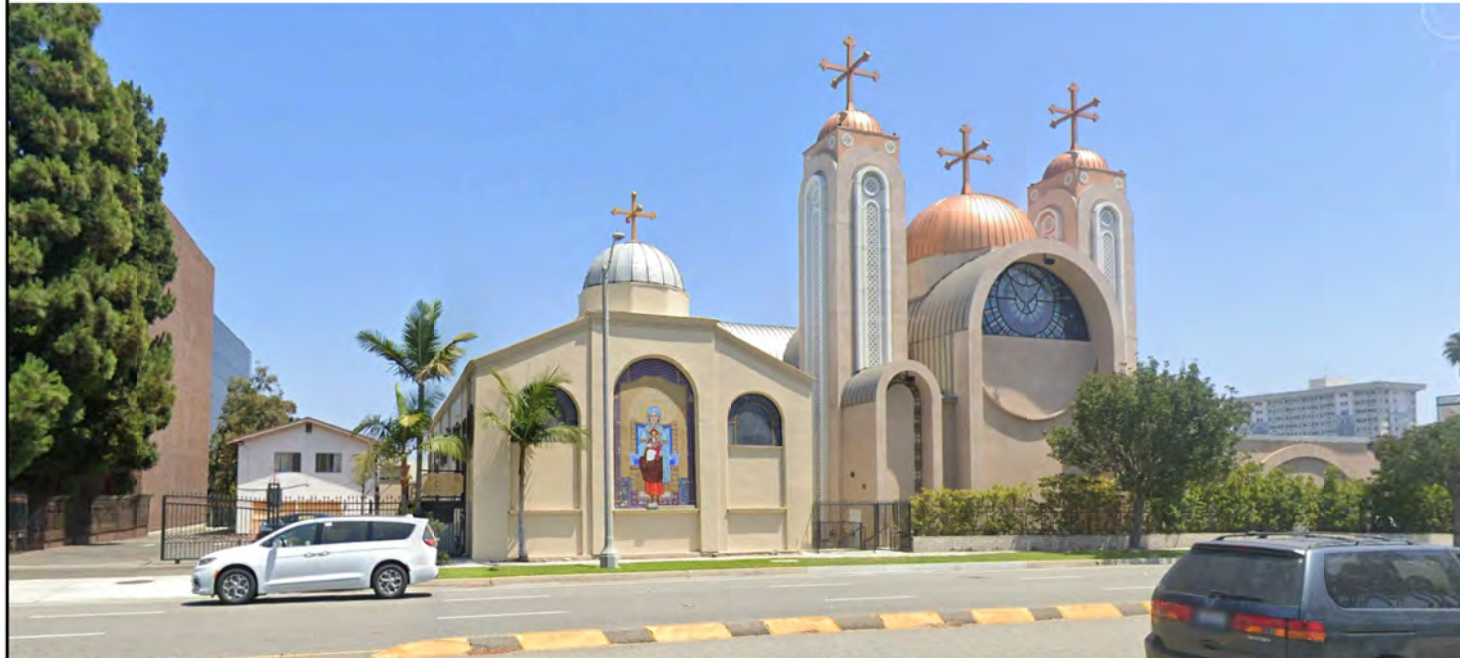
EXISTING SOUTH GROUND VIEW
