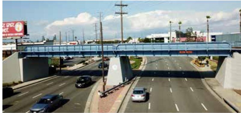
had no plans or projects to address the undesirable, rusty surface, Public Works staff proposed an alternative where the City would resurface (re-paint) the bridge via the services of a licensed contractor. LACMTA accepted our proposal and Public Works obtained a permit from LACMTA to resurface the bridge. The bridge resurfacing was completed in November 2023. Additionally, Public Works branded the bridge with two 3' diameter round city logo signs.
