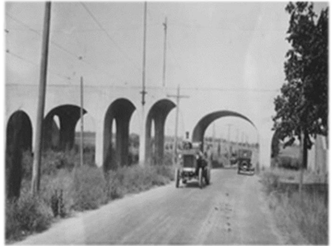
Figure 1: Pacific Electric Railway - El Prado Bridge
