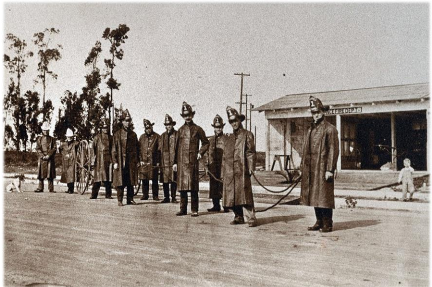
Figure 20: TFD Volunteer Fire Company - Two Wheeled Hose Cart
