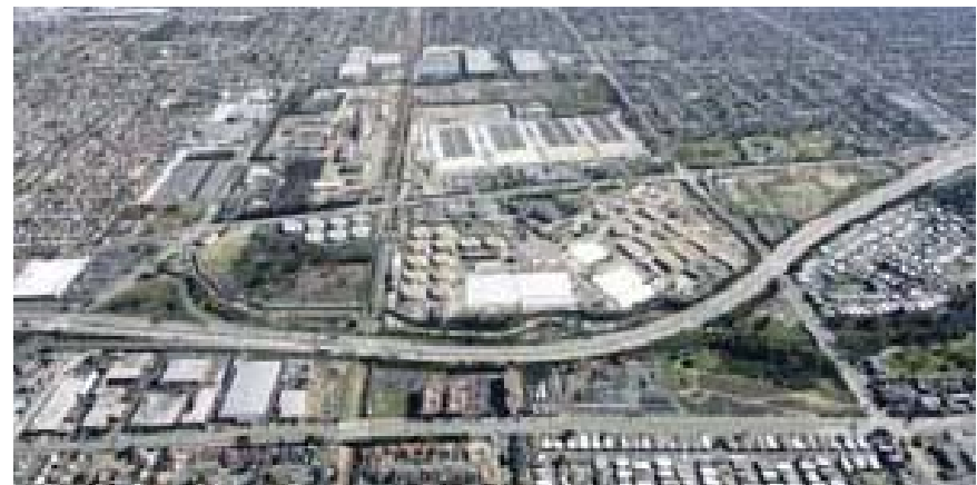
Joint Water Pollution Control Plant, Carson
