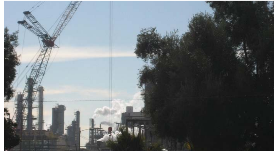
Exxon Mobile Refinery Source: The Planning Center, 2007
