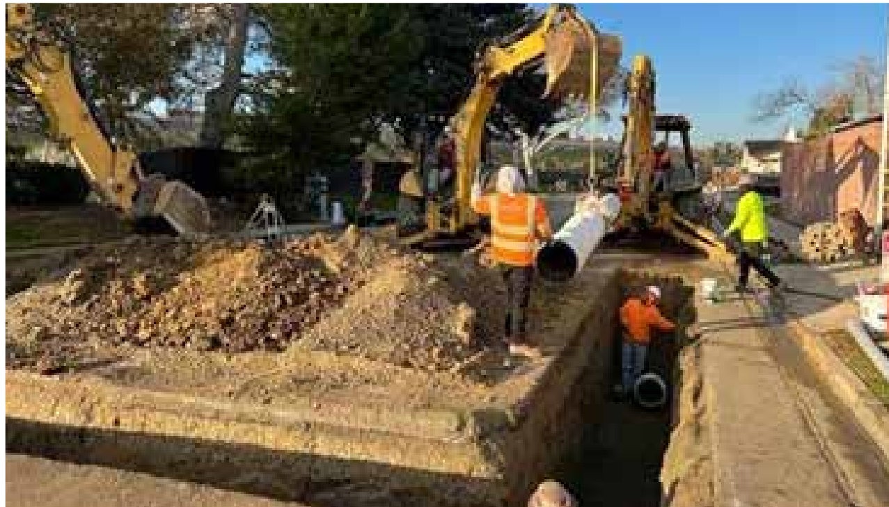
A crew works on installing new pipe.
