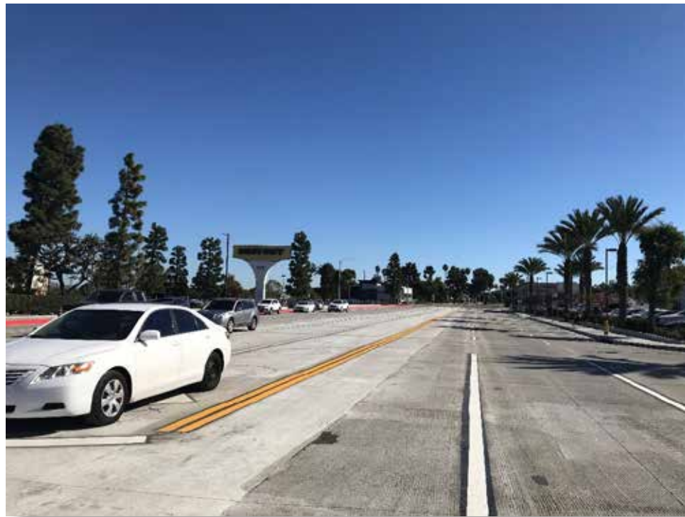
Completed concrete pavement and widened intersection looking east on Pacific Coast Highway.
