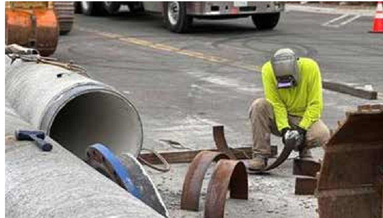
A worker prepares new transmission main pipe for installation.
