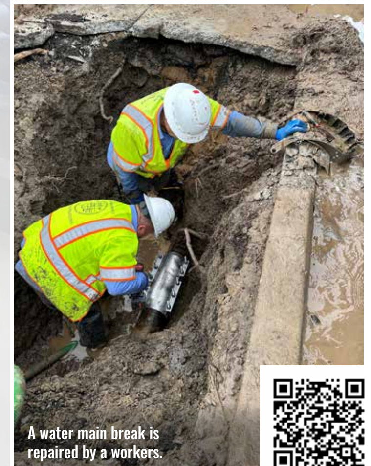
Water Operations staff connect residential service.
