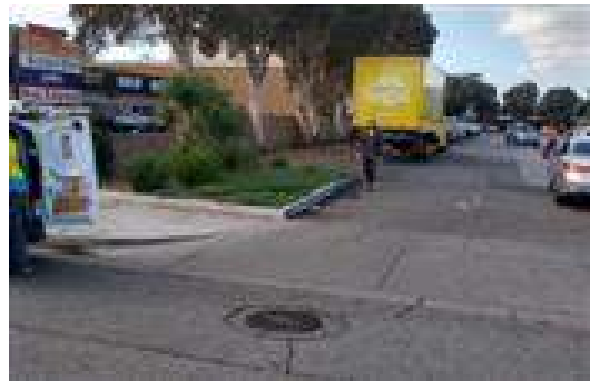
Manhole Before Install
