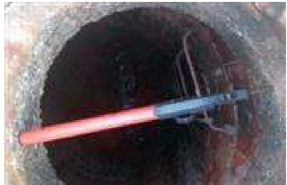
Manhole During Install
