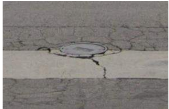
Manhole Before Install
