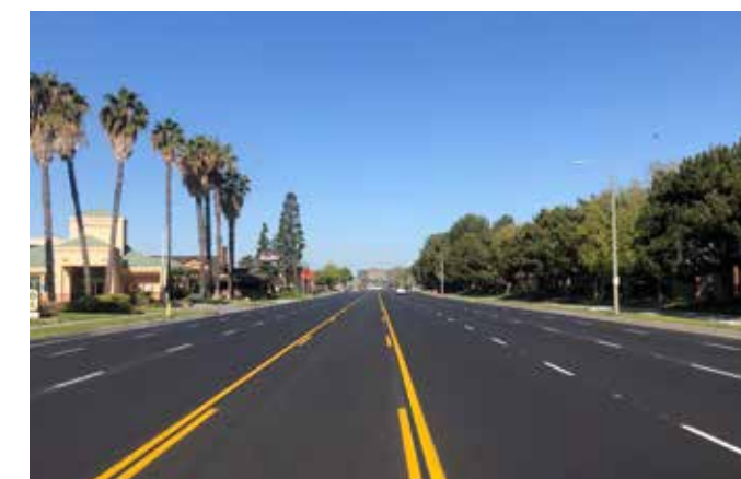
Sepulveda Boulevard looking west from Hickory Avenue
