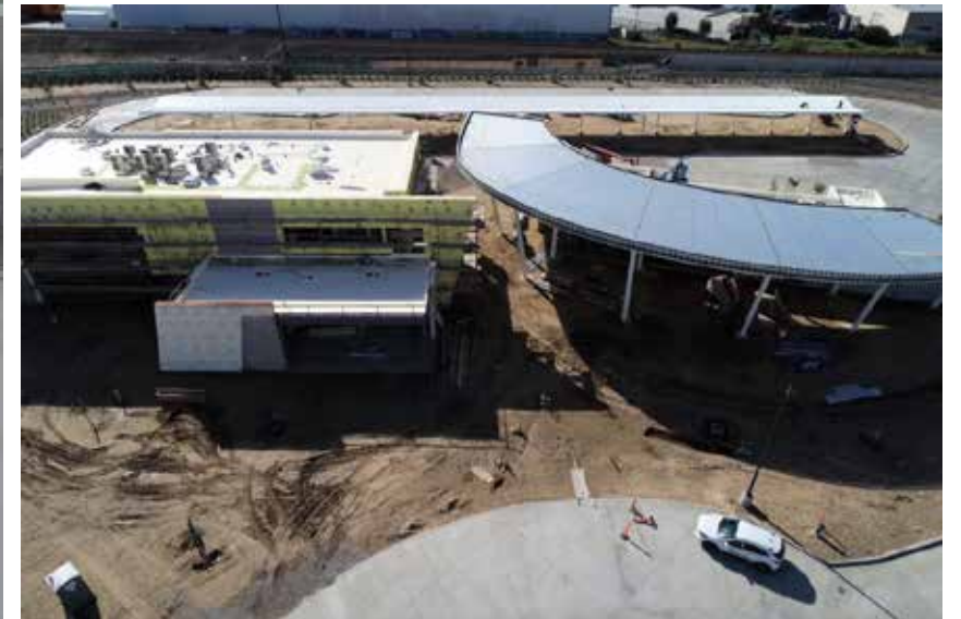
Aerial view of the Regional Transit Center under construction
