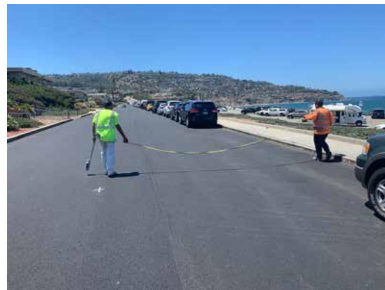
Measuring pavement for striping on Paseo de la Playa
