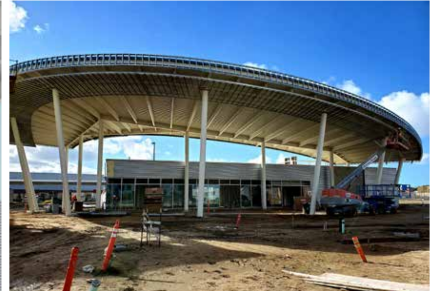
Regional Transit Center under construction
