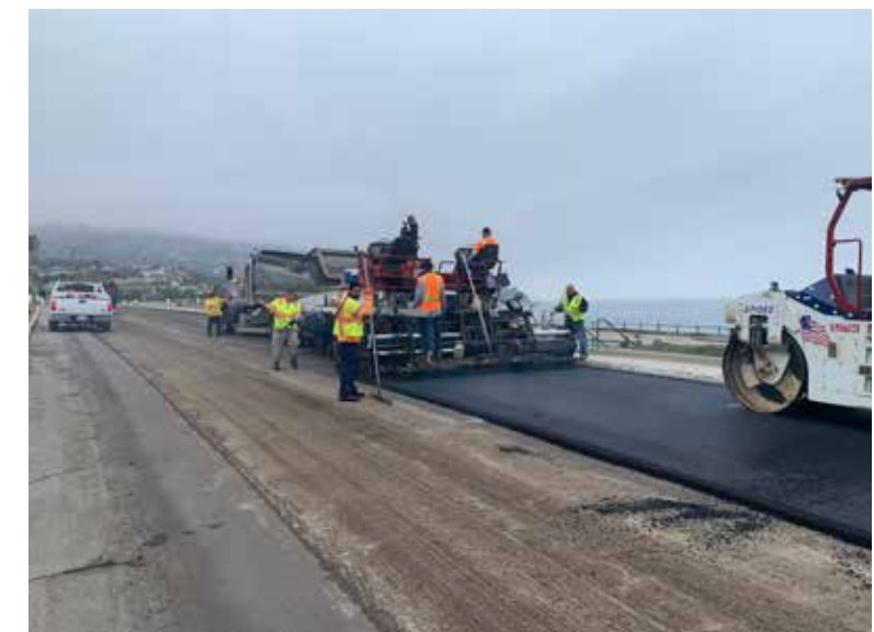
Paving operation on Paseo de la Playa
