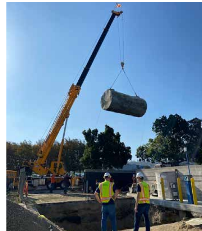
Underground storage tank removal
