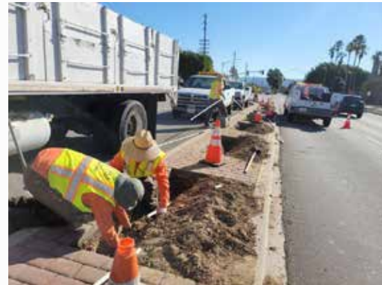
Landscape upgrades to center median - Madrona Avenue
