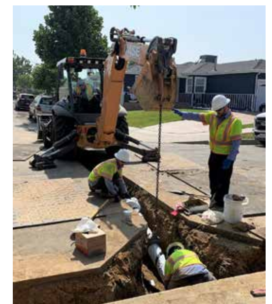
Water main installation
