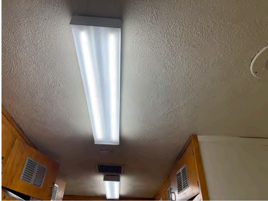
Non-asbestos textured ceiling plaster in hallway area.
