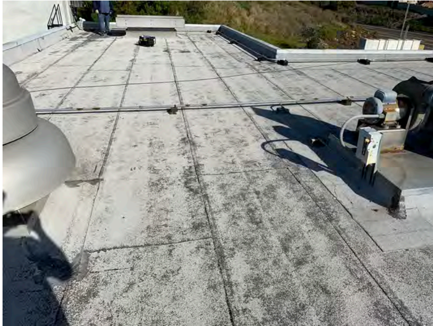
ACM flashing mastic and pedestal mastic – center roof.
