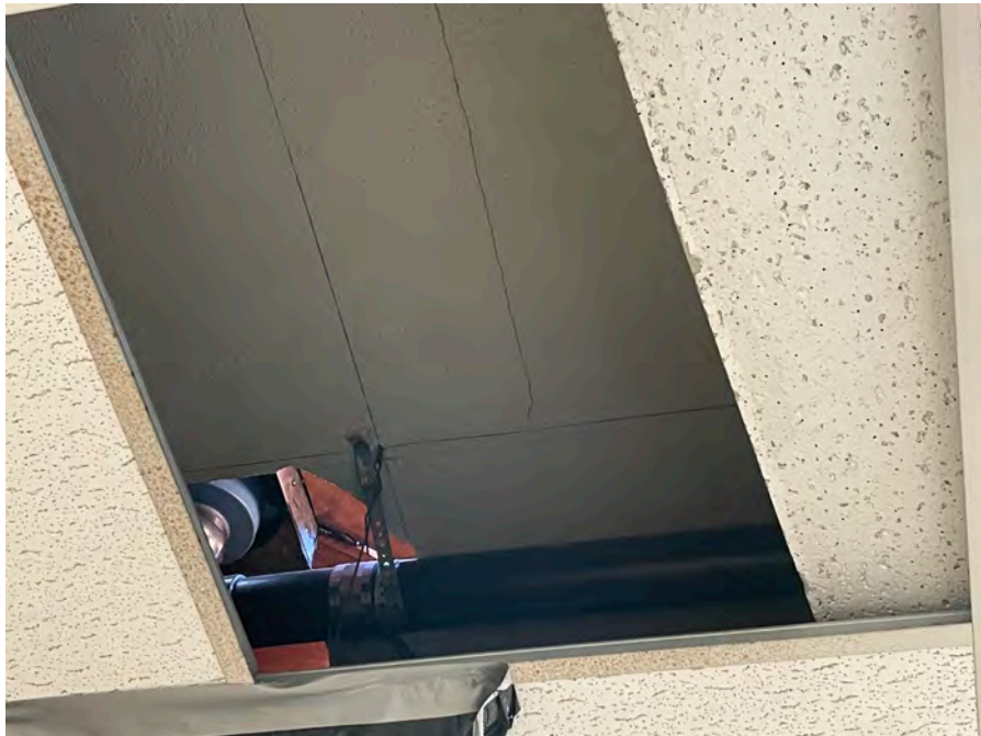
Non-asbestos textured ceiling plaster in subceiling space – dorm.
