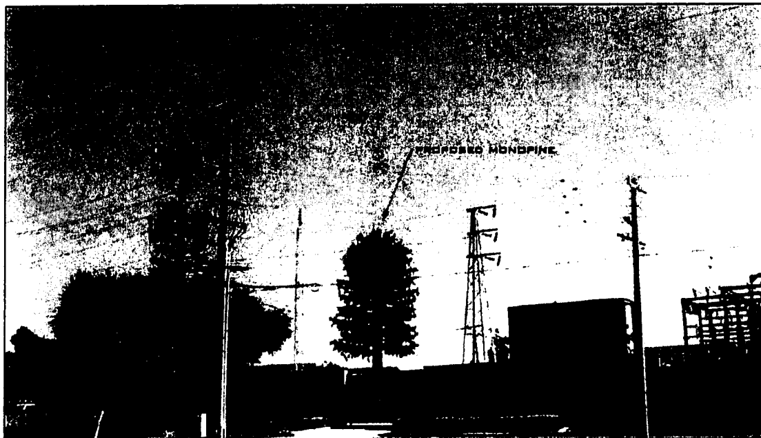
Figure 2: Photo simulation of proposed Monopine; annotations in original (Source: Applicant submitted Photo Simulations).
