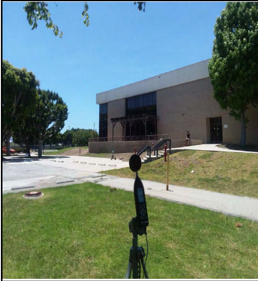
STNM1 looking SW towards SE corner of building, 2555 West 190th St, Torrance.
