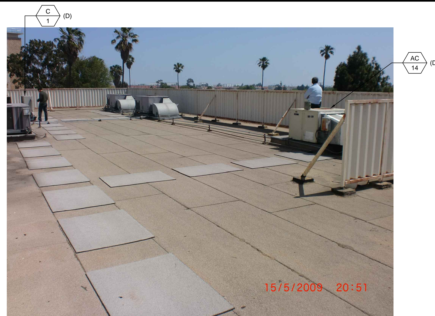
EXISTING UNITS ON ROOF NO SCALE 3
