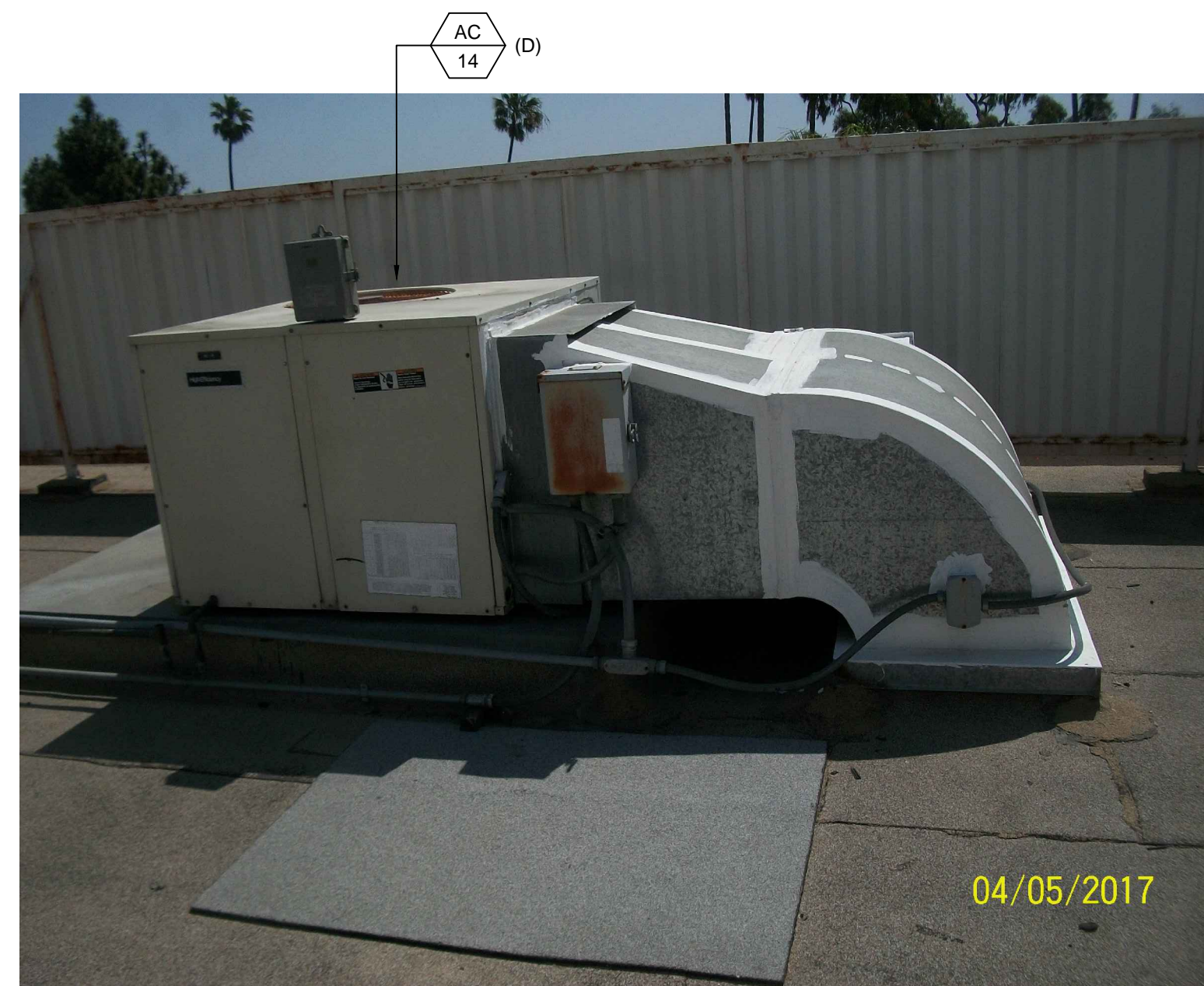
CONDENSER UNIT (TO BE DEMOLISHED) NO SCALE 5
