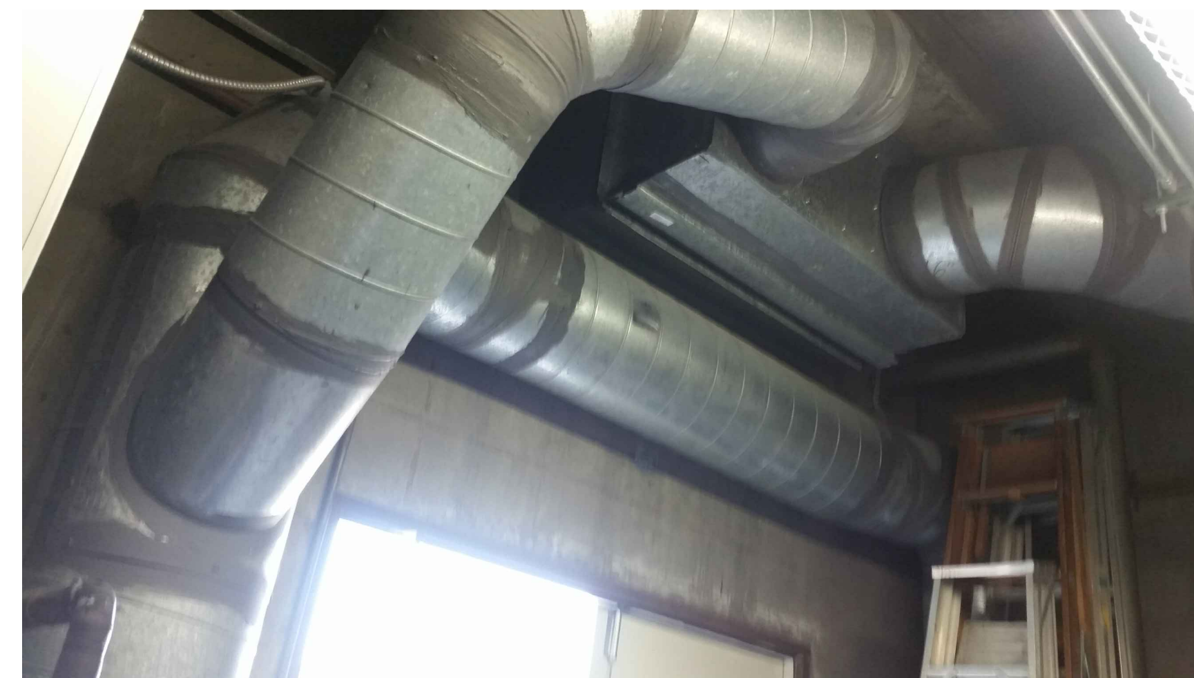
EXISTING OUTSIDE AIR INTAKE NO SCALE 2
