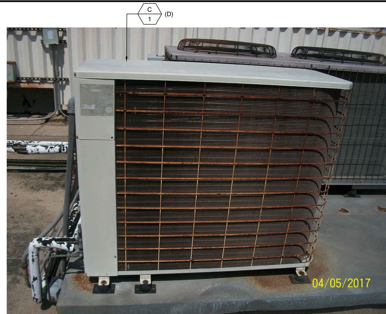
CONDENSER UNIT (TO BE DEMOLISHED) NO SCALE 5
