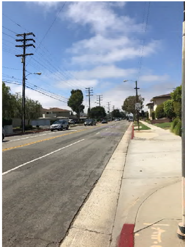
Overview of water main alignment on Van Ness Ave (view to SW)
