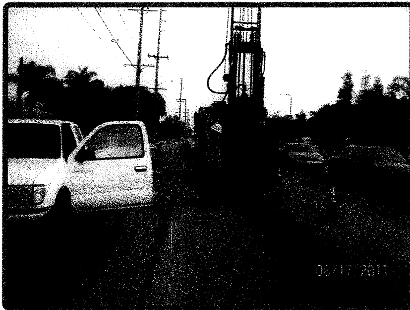
Photo 1: Photograph showing the drilling operations at soil boring location B-1 on Western Avenue in the City of Torrance, California.
