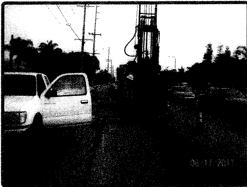
Photo 1: Photograph showing the drilling operations at soil boring location B-1 on Western Avenue in the City of Torrance, California.
