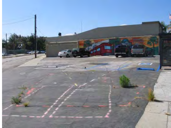
View Looking South
