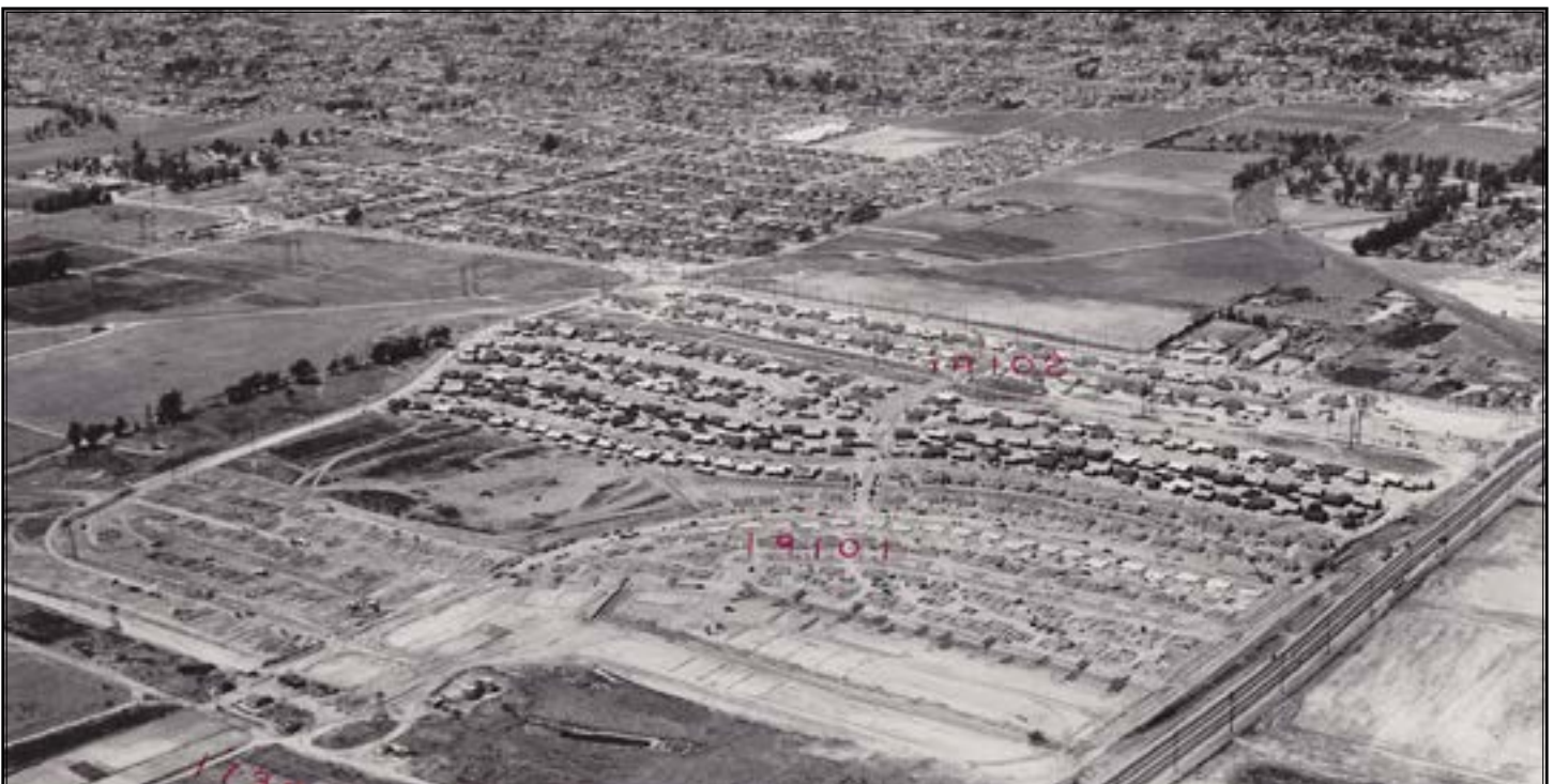
The Southwood tract at Sepulveda Boulevard west of Anza Avenue is seen during the construction phase in 1954.
