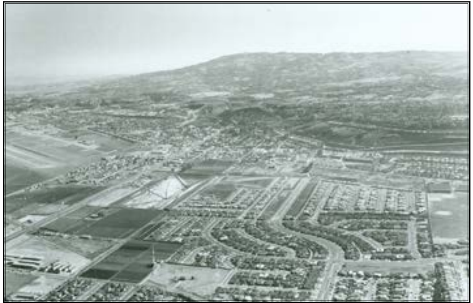
The Southwood Riviera Royale Development was a project by Don Wilson Builders. This image, from 1962, shows the project in the area of Anza Avenue and Calle Mayor.
