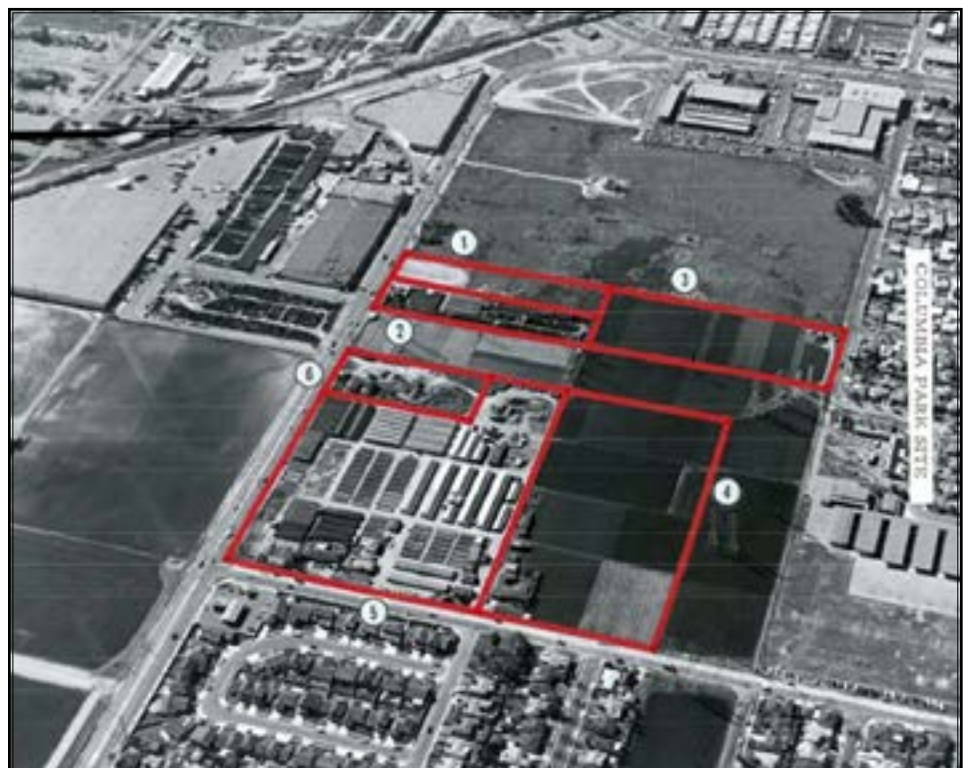
Columbia Park, a 50-acre park located at the corner of 190th Street and Prairie Avenue, was created through a partnership with the federal government, Los Angeles County, Southern California Edison, Columbia Broadcasting Company and the City.
