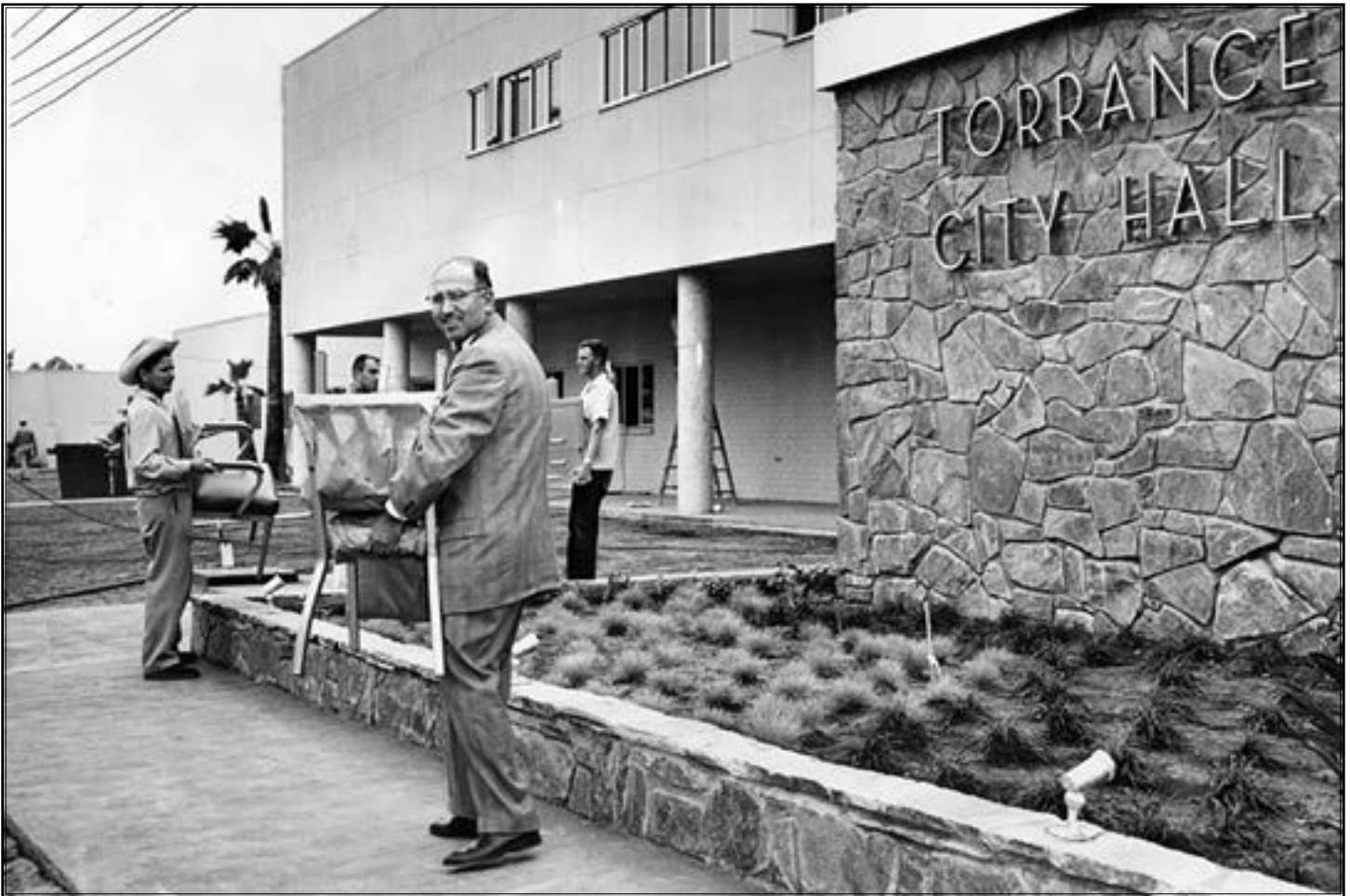
Torrance city officials moved into the new Civic Center in 1956. Mayor Albert Isen helped move furniture to his new offices. The Civic Center was built at a cost of $1,500,000.
