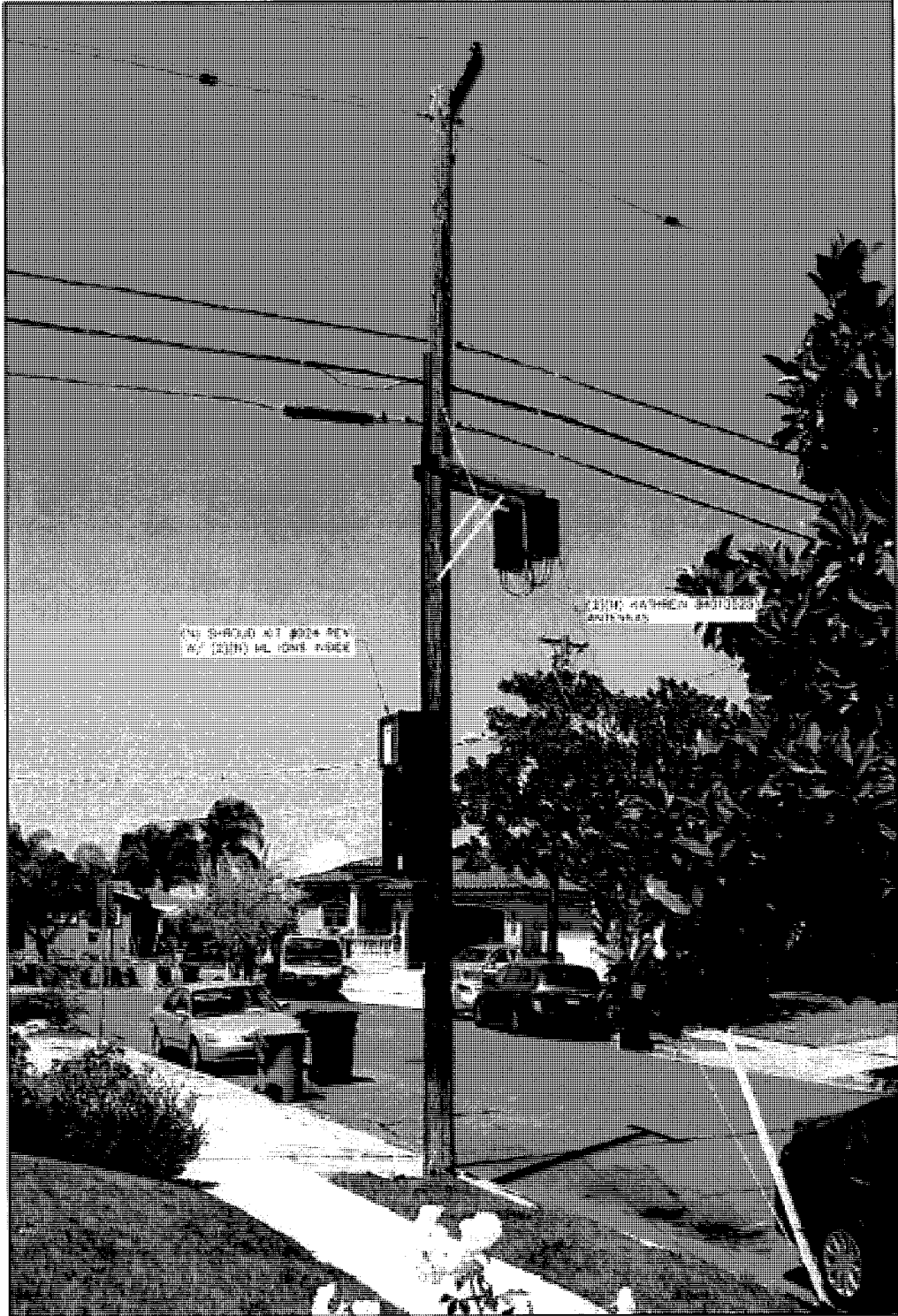
Figure 1: Proposed node on existing utility pole. (Source: Applicant's Photo Simulation provided by through its January 2018 Submission).
