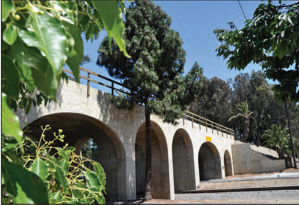
Pacific Electric Railway - El Prado Bridge
