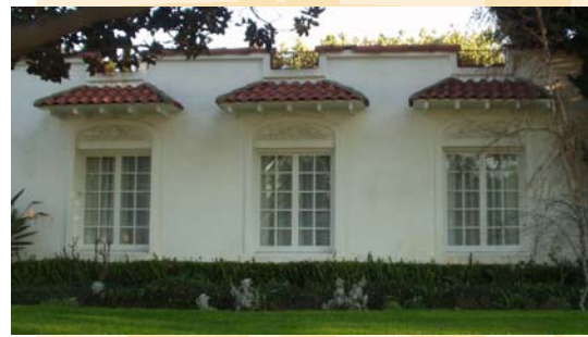
RED CLAY TILE ACCENTS & ROOF TRIM ON FLAT ROOF
