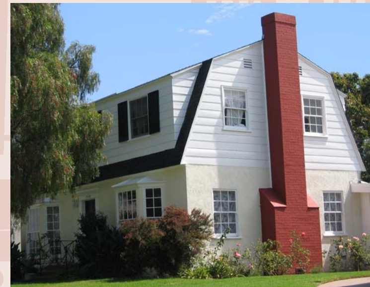
A DUTCH COLONIAL WITH STEEPLY PITCHED GAMBREL ROOF AND CONTINUOUS DORMER ACROSS FRONT ELEVATION
