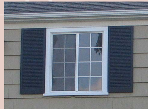
WOOD FRAMED WINDOW, WOOD SHUTTERS
