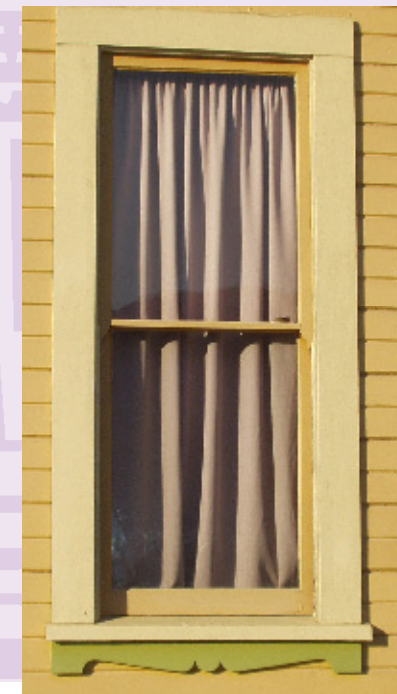
NARROW VICTORIAN STYLE WINDOW WITH ORNAMENTAL TRIM
