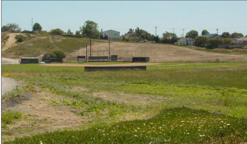
Detention Basin at Entradero Park: detention and retention basins (sumps) are scattered throughout the city that are used to store runoff
