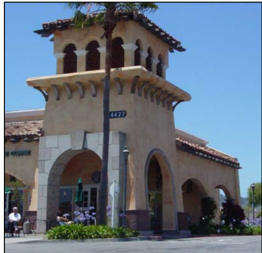
Torrance Crossroads Shopping Center: Attractive building and site design, extensive landscape treatments, and retailers and food establishments with a regional appeal have contributed to the success of the shopping center.
