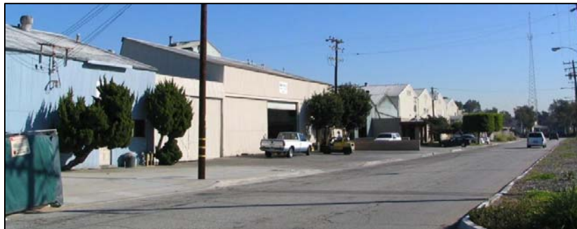
Jefferson/Oak: Industrial buildings along Jefferson Street located across from Wilson Park.
